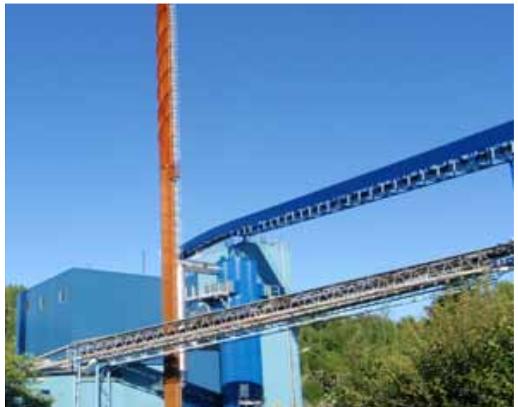
A biofuel boiler was brought into commission in 2010.
